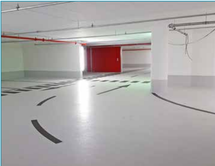
Fertige Beschichtung | Finished coating
