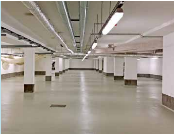
Fertige Beschichtung | Finished coating
