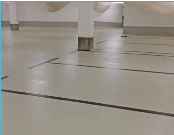
Fertige Beschichtung | Finished coating
