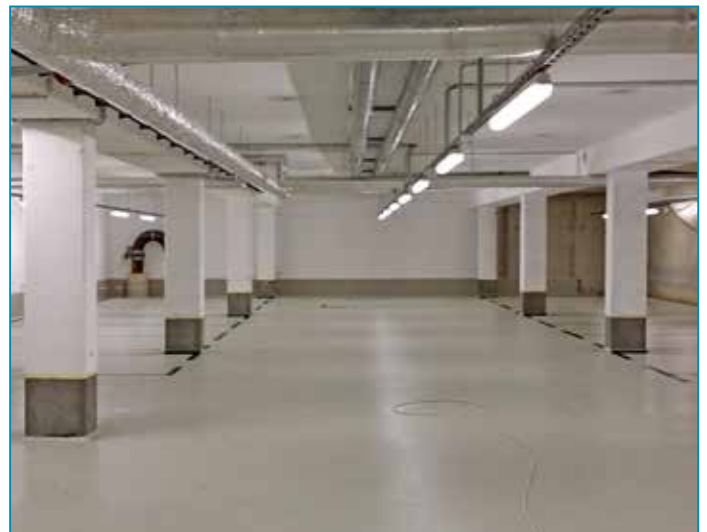
Fertige Beschichtung | Finished coating
