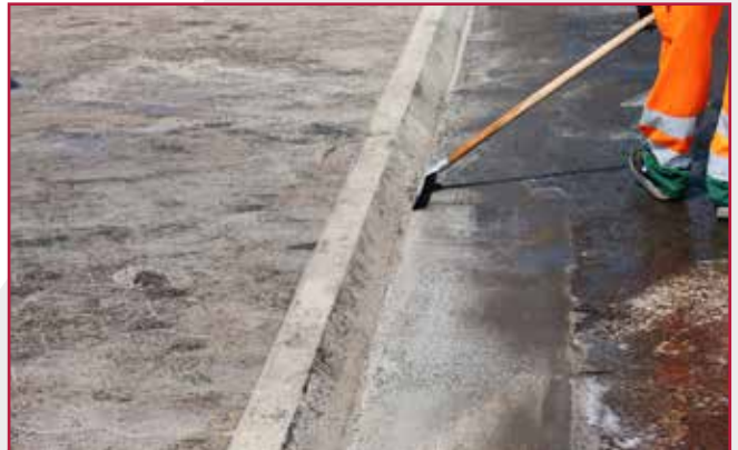
Die Randsteine inkl. der Fuge zur asphaltierten Straße wurden ebenfalls verschlossen The curbstones including the joints with the asphalt road, were also sealed
