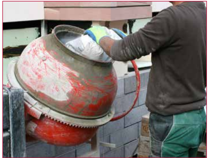
ROMEX® - TRASS-BETTUNG anmischen | ROMEX® - TRASS-BED being mixed
