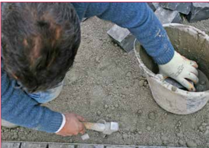
ROMEX® - TRASS-HAFTSCHLÄMME anwenden | ROMEX® - TRASS-ADHESION ELUTRIANTS being used
