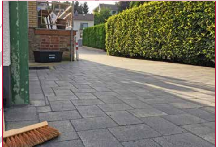
Abfegen-Endreinigung | Brush off – final cleaning
