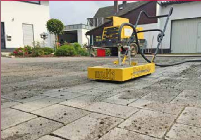
Reinigen der Altugen | Cleaning of old joints
