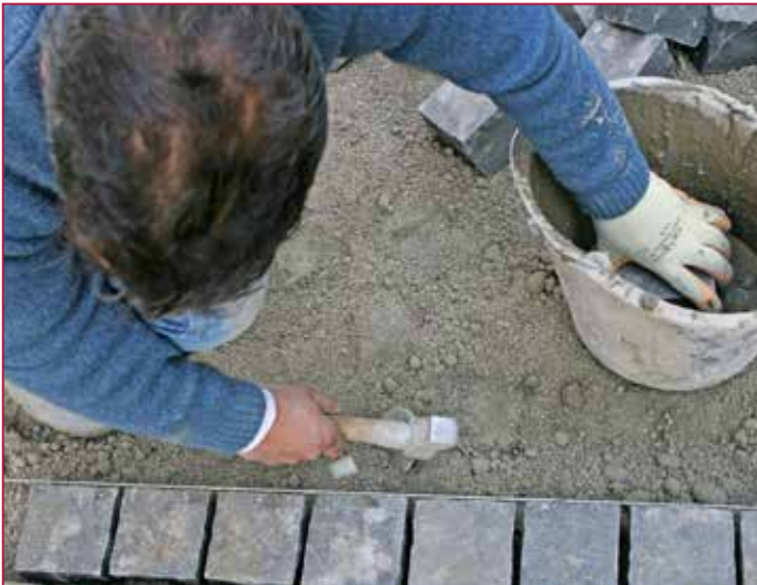
ROMEX® - TRASS-HAFTSCHLÄMME anwenden | ROMEX® - TRASS-ADHESION ELUTRIANTS being used
