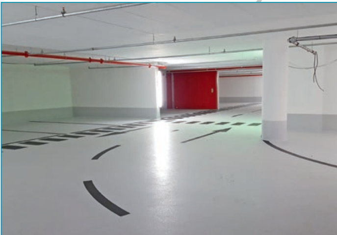
Fertige Beschichtung | Finished coating
