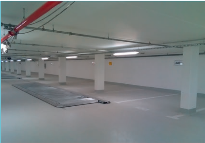
Mobiler Stellplatz | Mobile parking space
